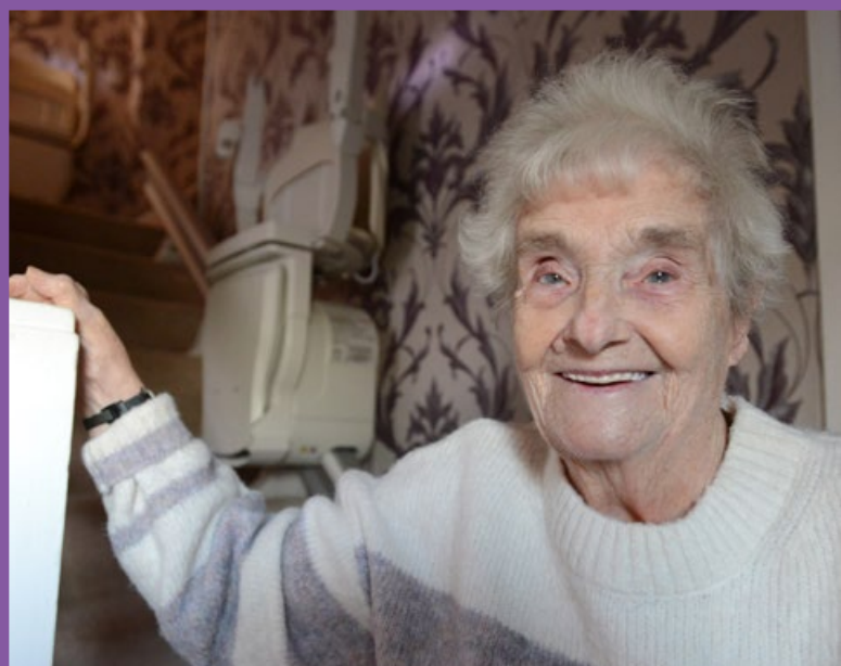
Local resident with a new stair lift installed by the See and Solve service
