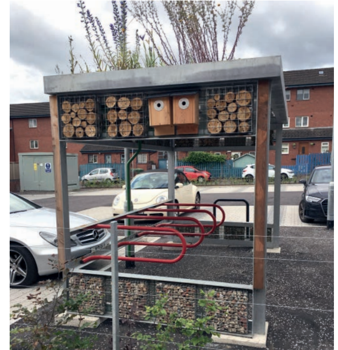
Figure 60: Bike shelter with habitat provision and green roof, serving commercial and multi-occupancy flat development, Glasgow
