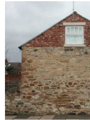
Rubble and brick wall
