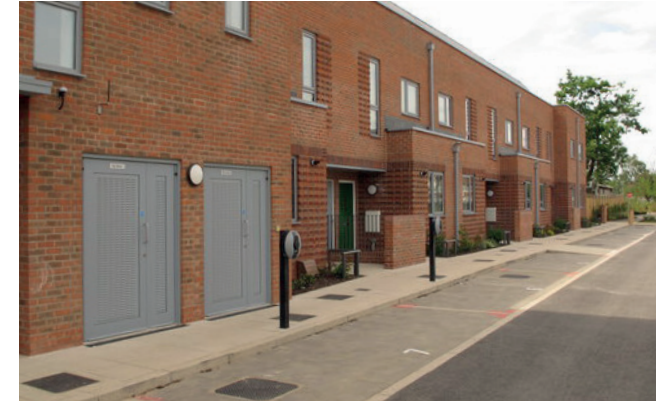
Figure 47: Electric charging points, North Acton
