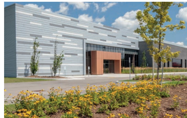
Figure 57: Industrial building at Hanlon Creek
