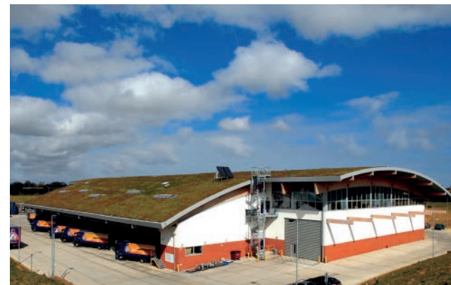
Figure 55: Green roof at the Adnams Distribution Centre
