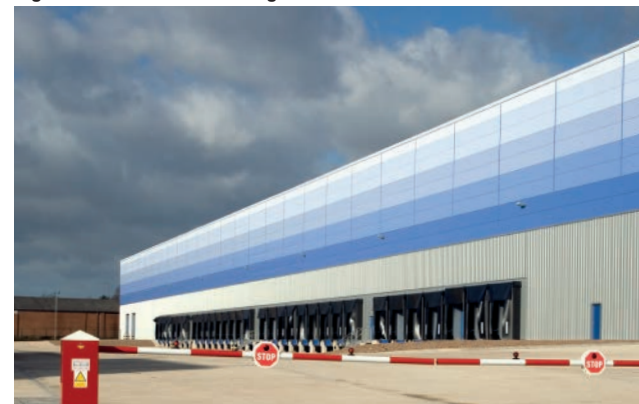
Figure 58: Blue panels designed to reduce visual impacts of industrial buildings at G Park, Workop
