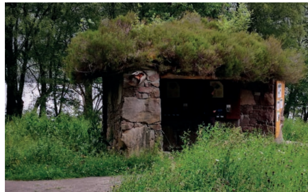
Figure 53: Green roof on information shelter, Highlands
