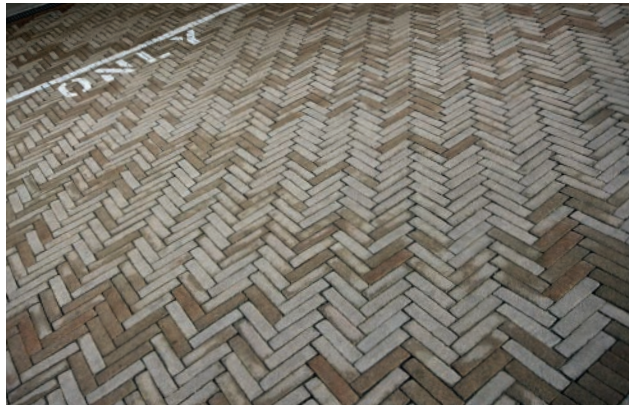
Figure 49: Permeable Paving (Hardscape)
