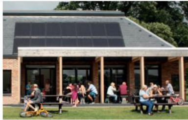
Figure 50: Solar Panels on a new build at Levensgrove Park, Dumbarton
