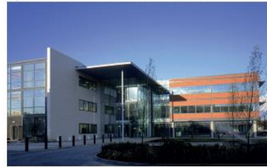
Figure 56: Windsor Business Park, Berkshire
