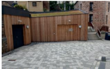
Figure 59: Large timber bin shelter with green roof for flats in Edinburgh
