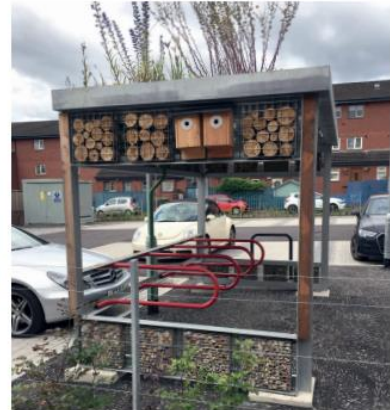
Figure 60: Bike shelter with habitat provision and green roof, serving commercial and multi-occupancy flat development, Glasgow
