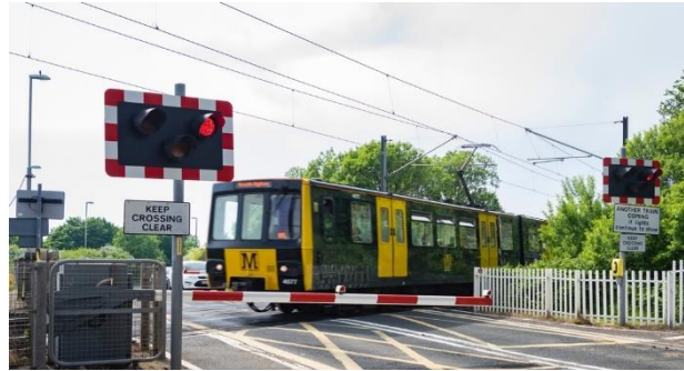
Figure 11: Tyne and Wear Metro at Tiledshed Lane Crossing
