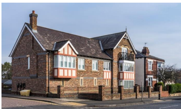
Figure 29: Front Street housing development
