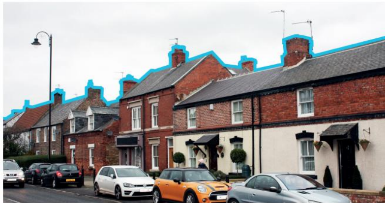
Figure 34: Varied roof line along Front Street
