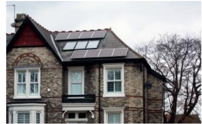
Figure 51: Example of retro-fitted solar panels in East Boldon
