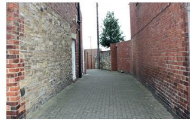
Figure 32: Narrow pedestrian passageways between Front Street and North Road
