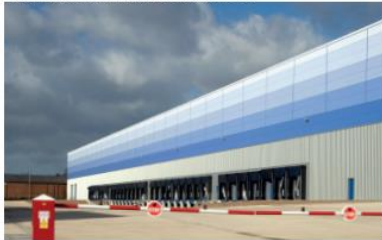
Figure 58: Blue panels designed to reduce visual impacts of industrial buildings at G Park, Workop
