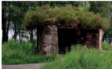
Figure 53: Green roof on information shelter, Highlands
