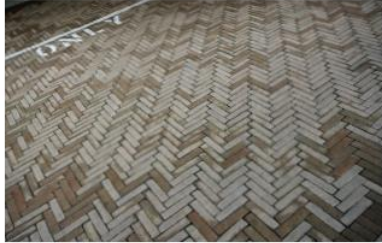
Figure 49: Permeable Paving (Hardscape)
