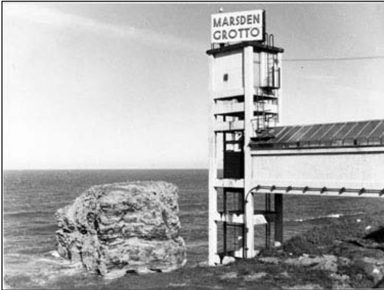
1956: Lift Shaft (photo courtesy of South Tyneside Libraries & Information)
