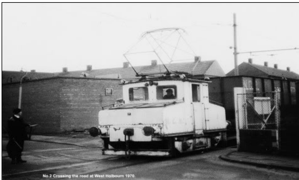
No.2 Crossing the road at West Holbourn 1970.
