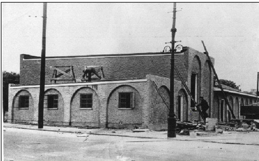
■ Converting the shelter to a theatre in 1948 ■
