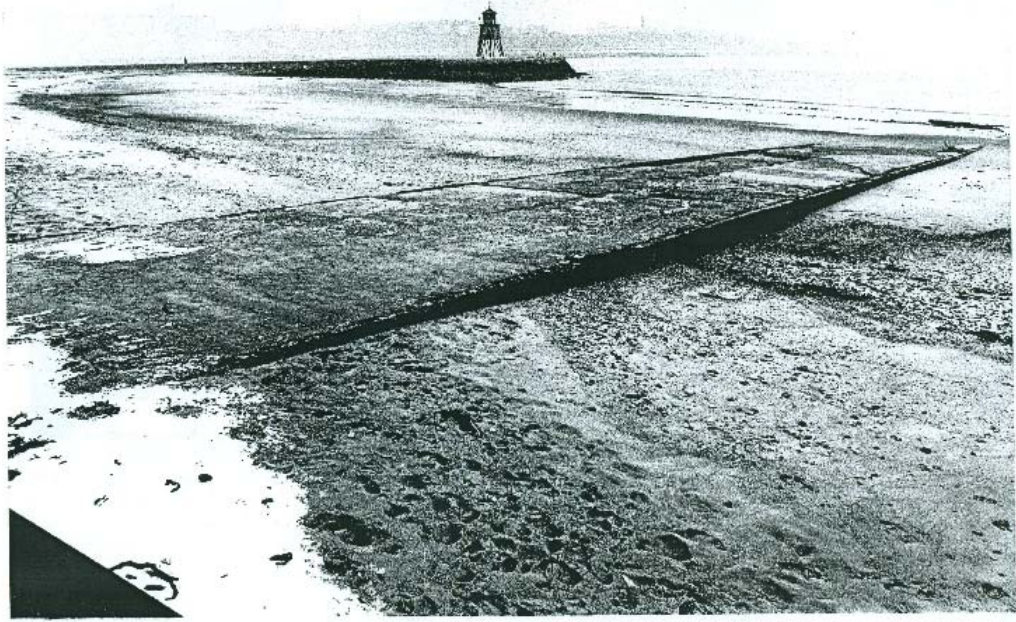
SEAPLANE SLIPWAY SOUTH SHIELDS
