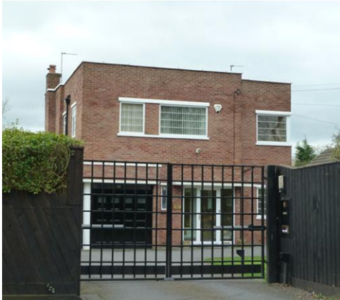
This Art Deco house was built in the 1930s in Cleadon. It displays the principal characteristics of a building of this type, with a flat roof, horizontal windows and windows cut through the wall returns. The building was recently restored and is particularly significant due to its rarity.
