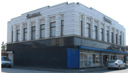
This impressive 1920s building was part of the Montague Burton tailoring empire. Montague was dedicated to providing high quality, made-to-measure suits at a reasonable price, revolutionising the industry. After the war the House of Burton produced a suit for war veterans nicknamed 'The Full Monty'.
