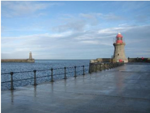
The foundation stones for both the North and South Piers were laid on 15 th June 1854 and a railway was constructed to carry the stones to the South Pier. Completed in 1895, the South Pier is 5170ft (1553m) long.
