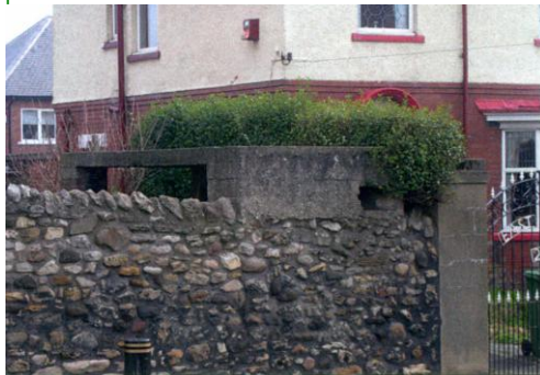
This Second World War pillbox has been built into an existing garden wall. A pillbox is a military bunker sited at a strategic point. They were hastily built all over the British Isles to defend against an anticipated German invasion.
