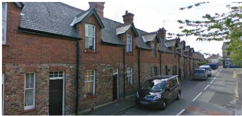
The one and a half storey cottages that make up Grange Terrace in East Boldon retain many of their original features, including sash windows and batted doors.
