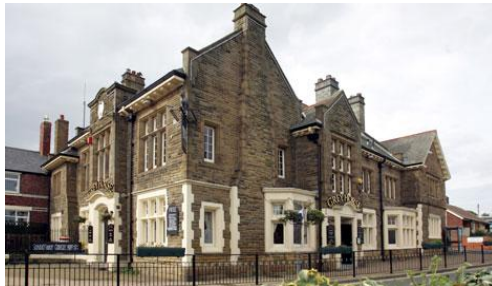
Grey Horse Public House (1905) is a prominent Tudor-gothic sandstone building with strong street presence.
