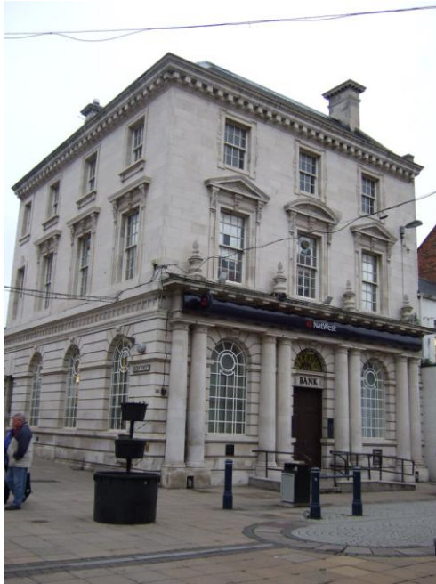
The Natwest Bank on King Street dates back to the 19 th century.
