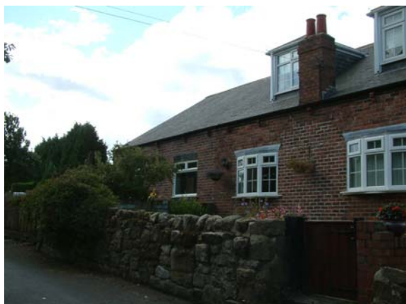
Figure 30 Brick cottage on Quay Corner Avenue, heavily altered. Simpson & Brown
