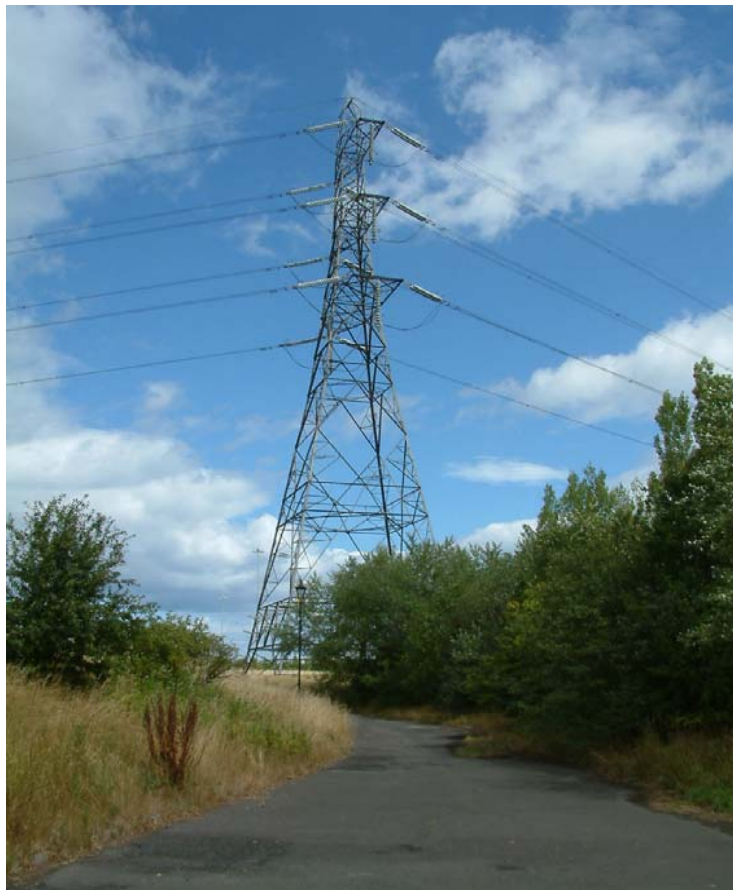
Figure 34 Cycle/pedestrian path and high voltage power lines. Simpson & Brown
