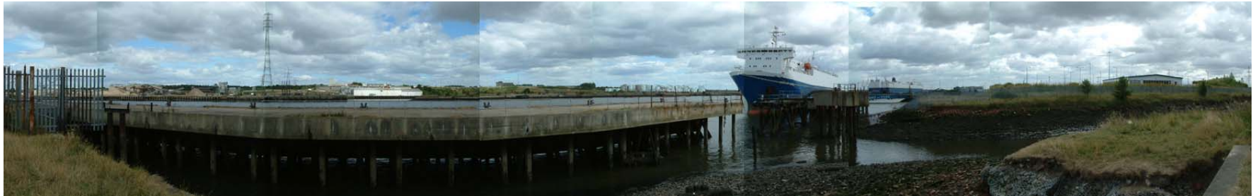
Figure 28 View looking northeast across the mouth of the River Don (right) and the River Tyne, showing the jetty and shipping use at the northernmost boundary of the conservation area. Simpson & Brown
