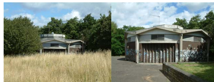
Figure 39 Don Valley Sewage Pumping Station in the south part of the conservation area. Simpson & Brown
