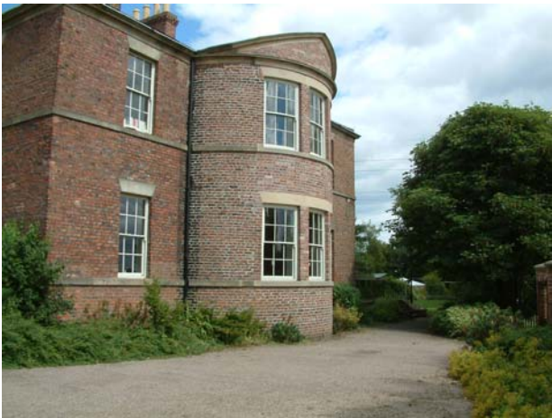
Figure 15 Jarrow Hall – brickwork. Simpson & Brown
