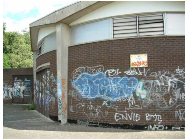
Figure 17 Don Valley Sewage Pumping Station, constructed in brick, concrete and steel. Simpson & Brown
