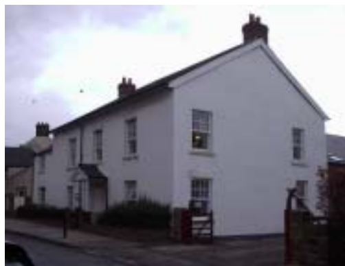
The White House (on the Local List), now a residential nursing home, comprises a large, simple, mid to late-nineteenth century house and a large late-twentieth century
