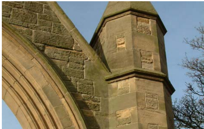
Figure 17 Sandstone of the Hebburn Cemetery entrance gate. Simpson & Brown
