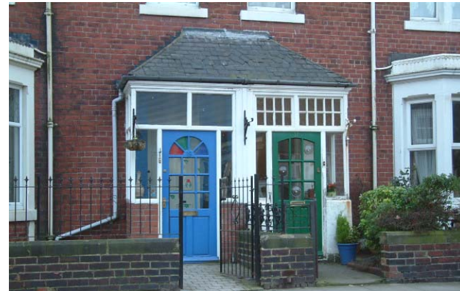
Figure 18 Brick and painted detailing of terrace housing. Simpson & Brown
