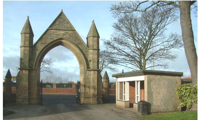
Figure 49 Intrusive shelter structure inside entrance gates to Hebburn Cemetery. Simpson & Brown
