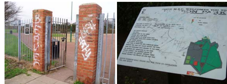
Figure 40 Graffiti on gate piers and vandalised interpretations sign. Simpson & Brown
