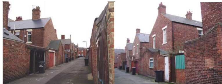
Figure 42 The form and character of back lanes remains largely intact. Simpson & Brown
