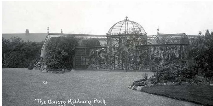
Figure 12 Late 19 th /early 20 th century aviary northeast of Hebburn Hall, demolished by the 1940s. National Monument Record – English Heritage
