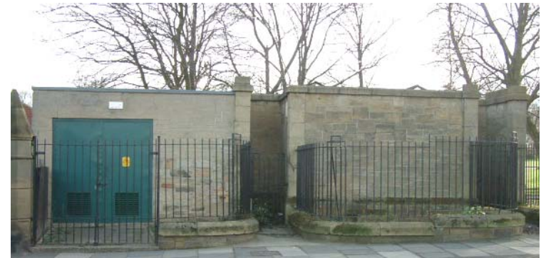
Figure 48 Electricity substation and toilet block. Simpson & Brown
