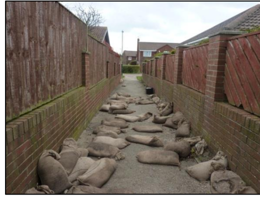
Photograph 6: Flow route into the residential area
