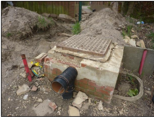
Photograph 3: Inlet to NWL storm sewer north of the estate
