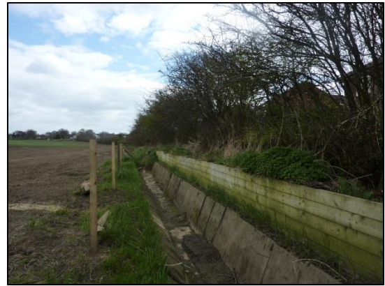
Photograph 4: Existing defence asset to manage surface water runoff
