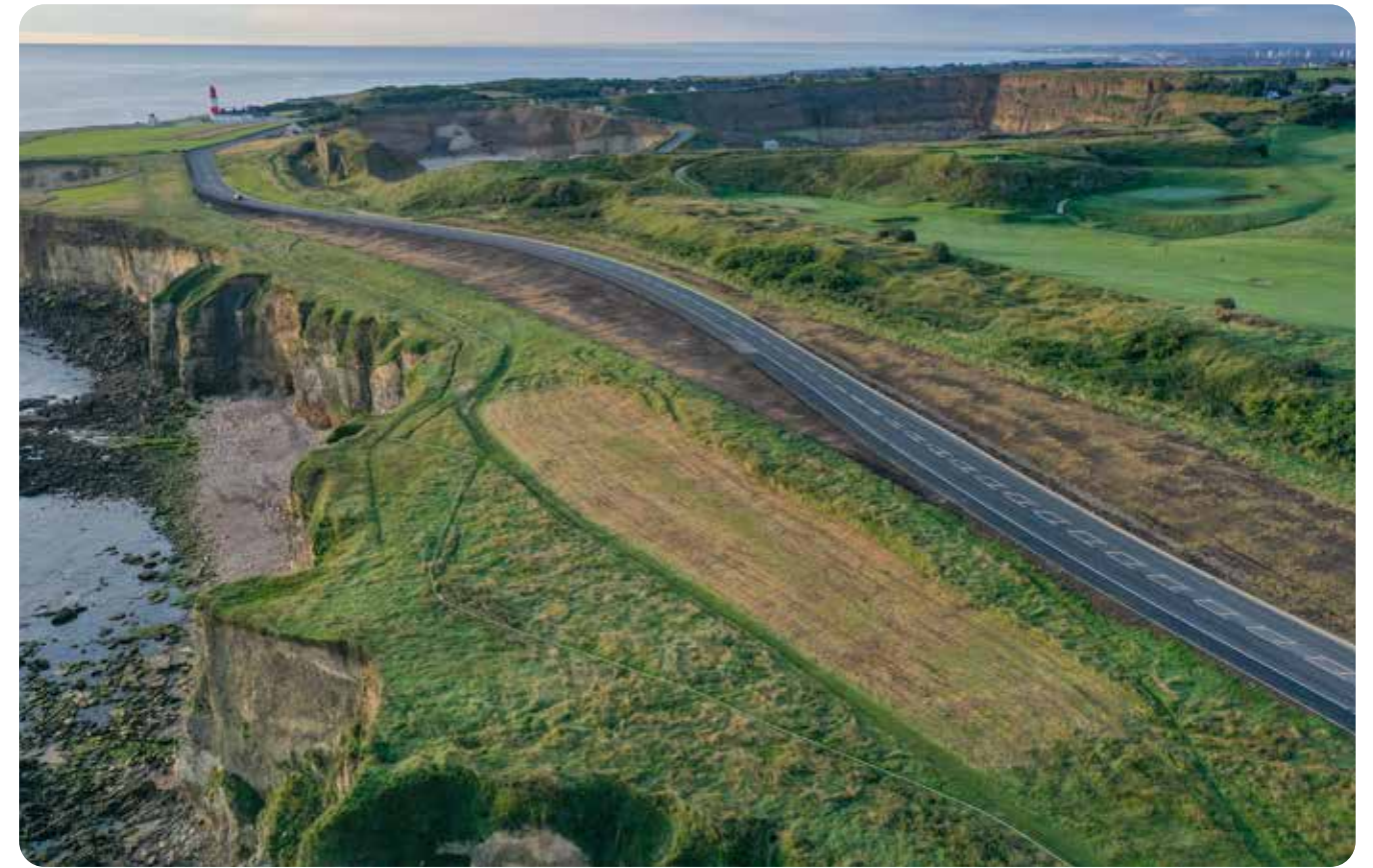
Completed coast road alignment works
