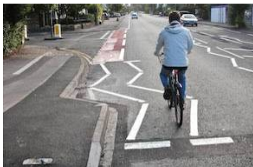
This example from another Region demonstrates that unsympathetically designed cycle lanes can not only look unsightly but can create conflict with other road users, sometimes generating dangerous situations for cyclists.
