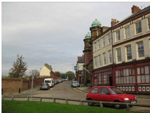
The introduction of an active frontage to the west side of Mill Dam Road could considerably enhance the Conservation Area provided that historic structures are acknowledged in any development proposal.
