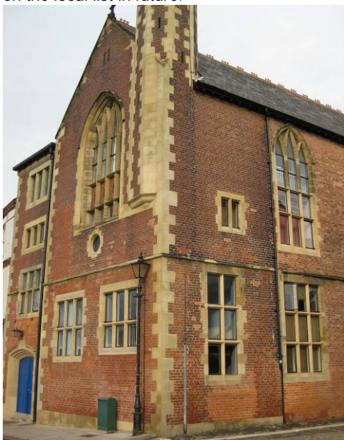
Unity Hall's strong Gothicised vertical form with asymmetrical gable and bell tower are emphasised by a high first floor tracery window. Stone moulding and quoins contribute to its authentic character.
