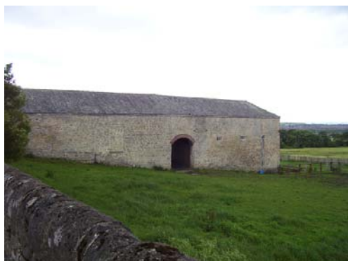
The group of buildings that form Sunnyside Farm have few external openings. Conversion would be challenging and could be harmful to the character and appearance of the Conservation Area.
