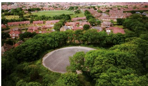
The concrete domed reservoir is redundant and could easily fall into disrepair.
