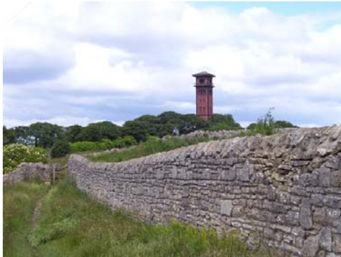
Magnesian limestone walls form the boundary of Cleadon Hills Local Nature Reserve and adjacent farmland
