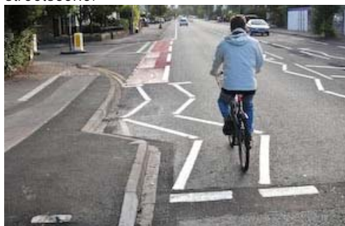
This example from another Region demonstrates that cycle lanes can not only look unsightly but can create conflict with other road users, sometimes generating dangerous situations for cyclists.
