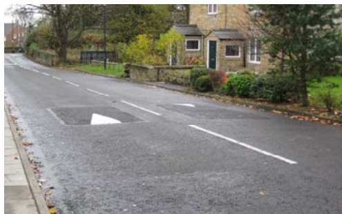
A lack of signage and minimal road markings lessen the impact of these speed cushions on the character and appearance of the streetscene.
