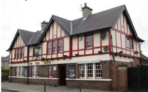
The Lord Nelson Public House is a unique building, full of character. It could potentially qualify for inclusion on the local list in future.
