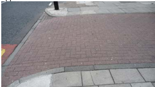
Using standard asphalt as an alternative surface treatment would avoid the introduction of too many different materials.
