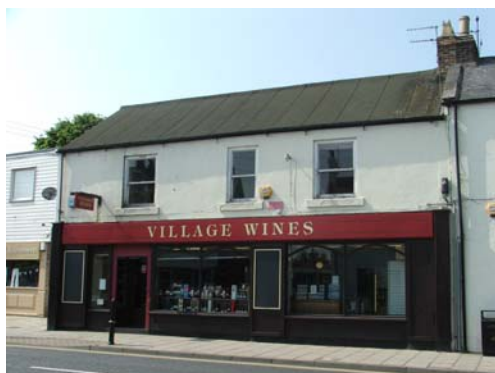
This shopfront sweeps across the ground floor of two Nineteenth Century buildings. It would have been more sympathetic to respect the individual plot widths.
