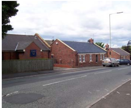
The Parish Hall lies at the summit of North Road and is a pivotal building within the community
