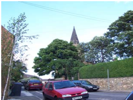
St. Nicholas Church is Grade I listed and a prominent local landmark
