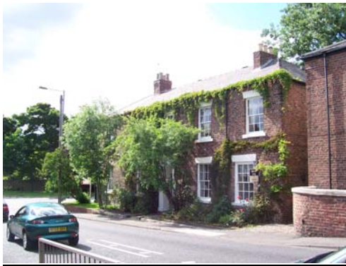
The A184 passes through the village centre and is a busy artery between Newcastle and Sunderland
