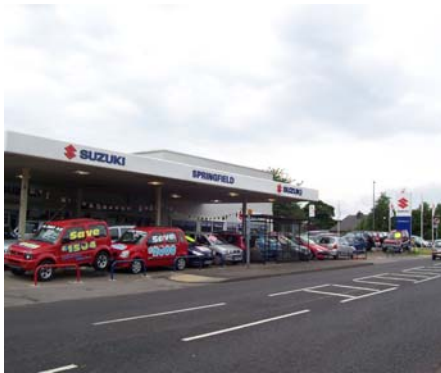
Bank Top Garage before closure
