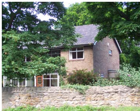
Sections of Newcastle Road are characterised by detached dwellings set back from historic boundary walls
