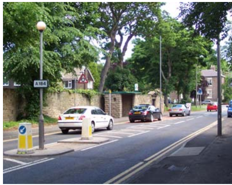
Street furniture and road markings make a significant impact on the character of the Conservation Area
