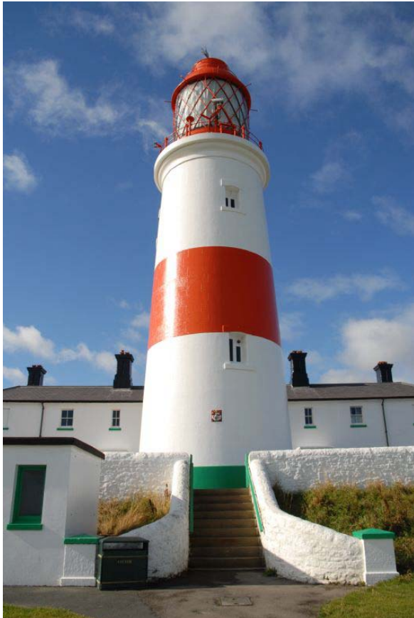
Above: the Grade II Listed Souter Lighthouse
