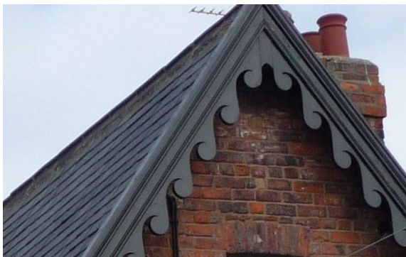
Timber eaves details add interest to a property.
