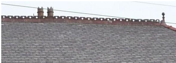
Traditional terracotta ridge detailing to a roof covered in Welsh slate.
