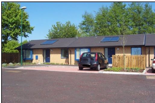
Residential car parking at Lavender Lane, West Harton
