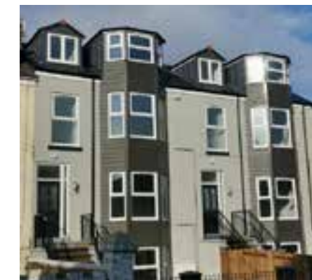
Eyesore building on Beach Road transformed into apartments for affordable rent
