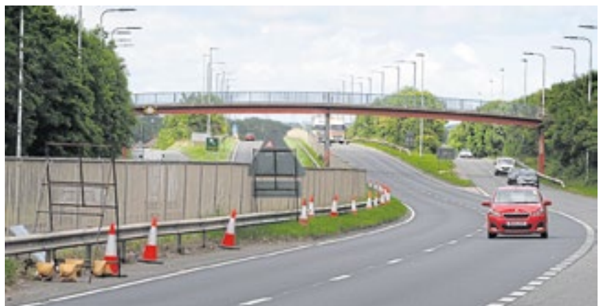
Kirkstone Avenue footbridge
