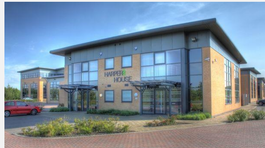
Figure 5.6: example of self contained office unit
