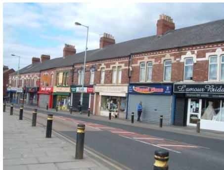
Top to bottom: Harton Nook, Frederick Street and Boldon Lane District Shopping Centres
