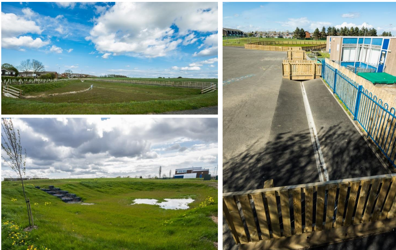
Figure 2: Some of the Fellgate Flood Alleviation Scheme SUDS Features
