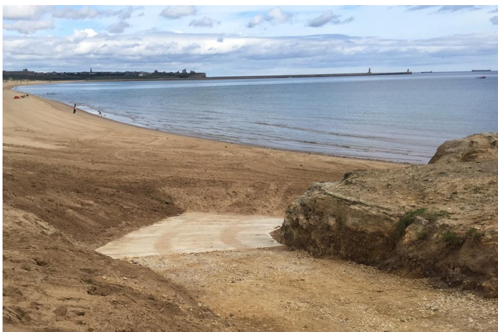
Figure 4 Herd Sands Access Ramp and Gabions
